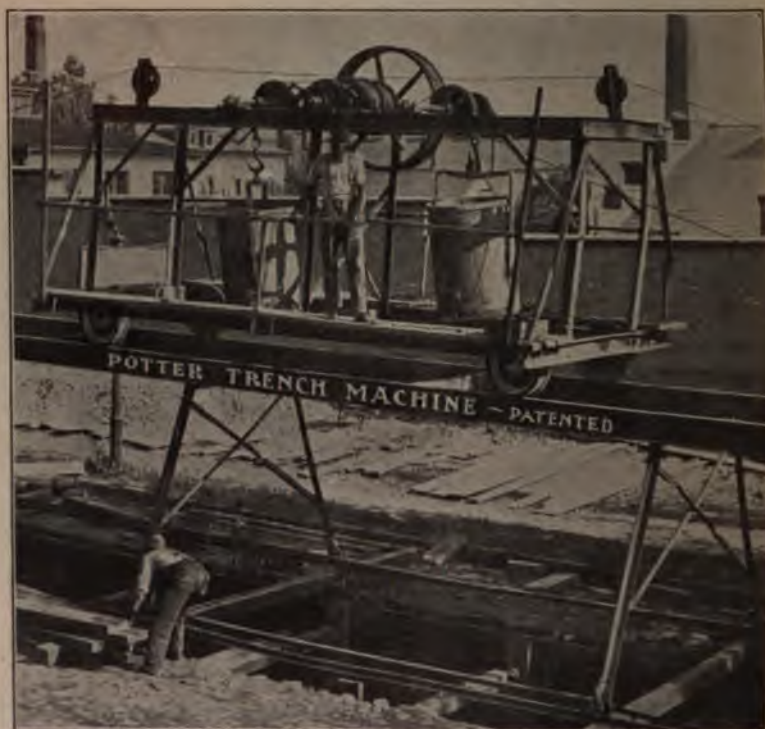
Trestle Track Excavator. Figure 124.
